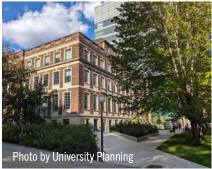
2024 | FitzGerald Building Revitalization
