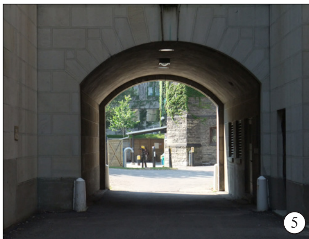
View through Canadiana Building walkway towards site
