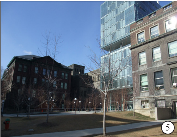
CCBR, Mining and Rosebrugh Buildings
