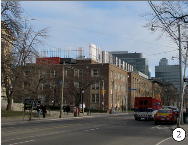
Wallberg Building; view east along College Street
