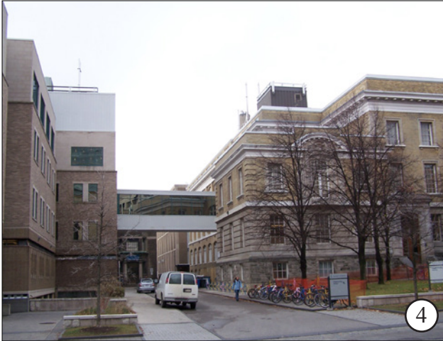
View west between Pratt and Sanford Fleming Buildings
