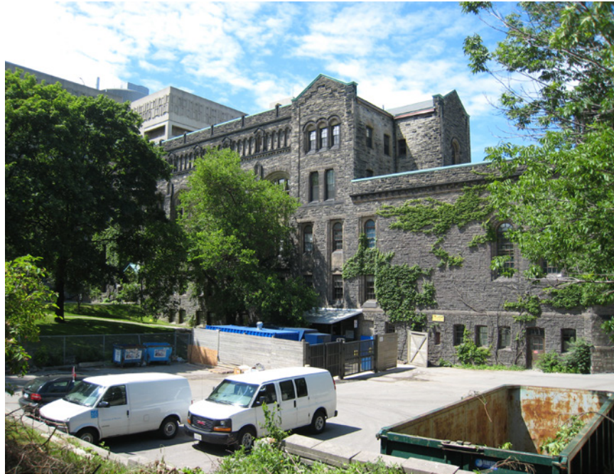
West side of Queen's Park Crescent (McMurrich Building)
