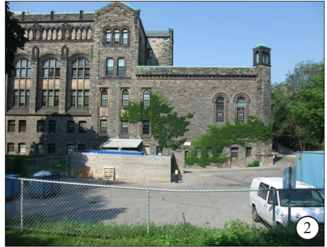
McMurrich Building existing service court (development site)
