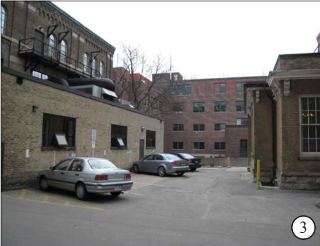
View south between Engineering Annex and Cumberland House
