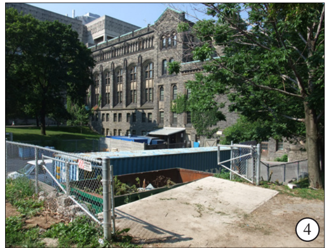
East facade of McMurrich Building
