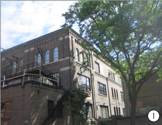
Engineering Annex; west facade
