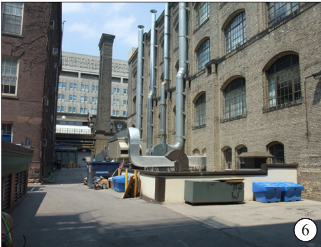
Haultain Building loading and mechanical spaces
