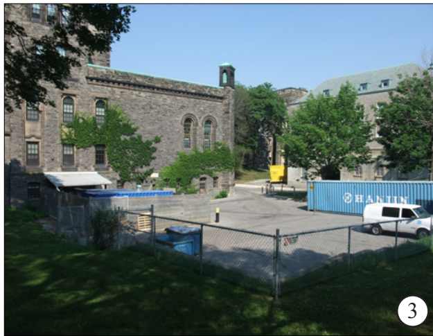
Existing service court, northwest view
