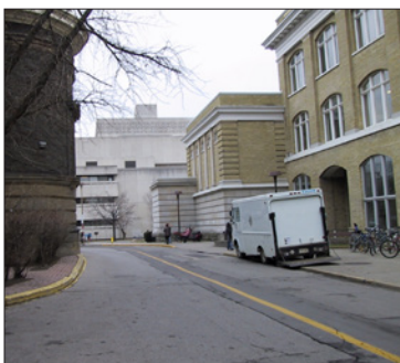
Existing service laneways are heavily used by the University community as secondary pedestrian environments.
