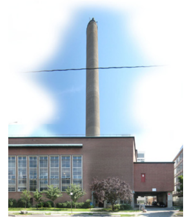
The Central Steam Plant is located in the south-west quadrant of campus
