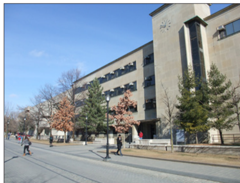
Mechanical Engineering, West Building, 1948. Listed. (above)
