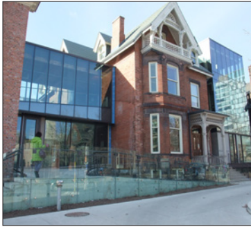
Department of Economics' new ramp; a design feature of the recent expansion
