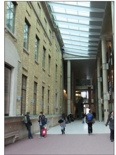
The Bahen Centre for Information Technology was constructed with an atrium that highlights the north heritage facade of the Koffler Student Centre, while providing access and connections between the two buildings.
