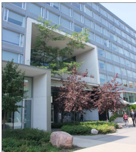
Woodsworth College Residence, courtyard (far left)
