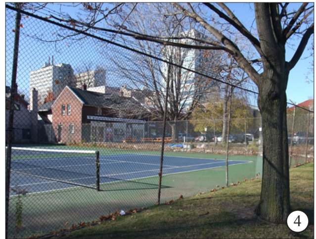
Trinity College's tennis courts to remain; Annex building beyond to be demolished
