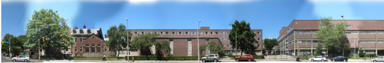
North side of Wellesley Street
