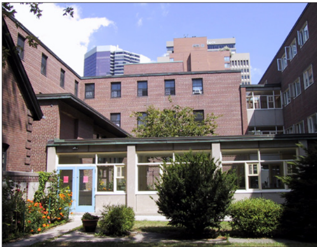
Connection between 74 and 90 Wellesley Street W
