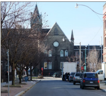
One Spadina east facade from Russell Street
