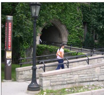
Accessible entrance to Hart House
